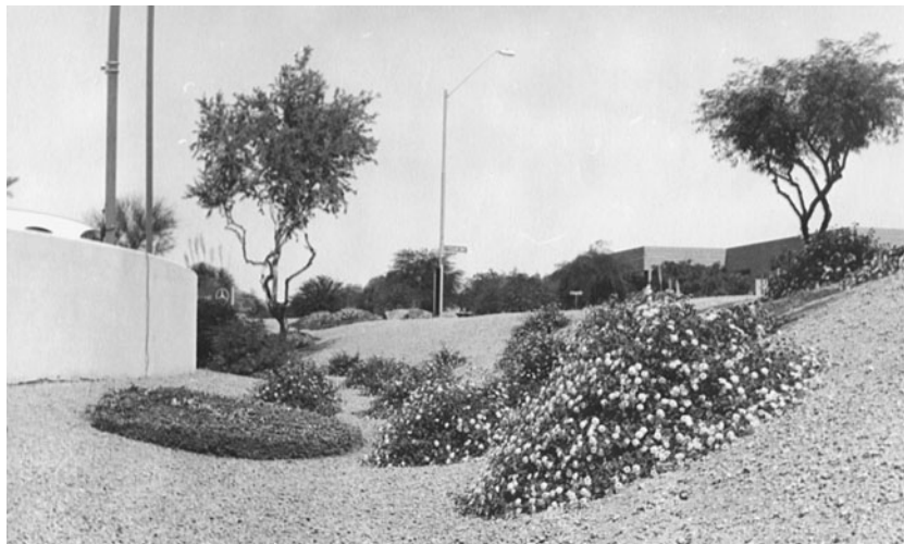
Figure 10.3 Small commercial lot detention facility.
